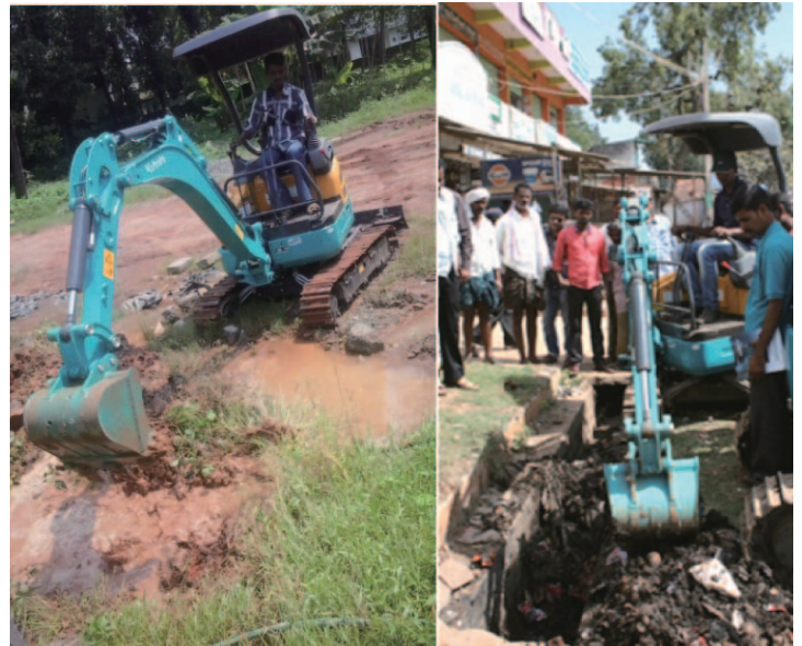
■ Canal / Drainage canal cleaning
